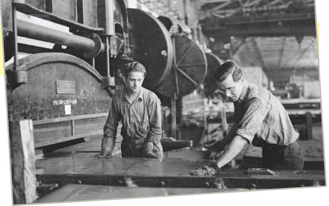
Worker cutting steel sheets, Pittsburgh, 1938. Courtesy of Farm Security Administration-Office of War Information Photograph Collections, Prints and Photographs Division, Library of Congress.
